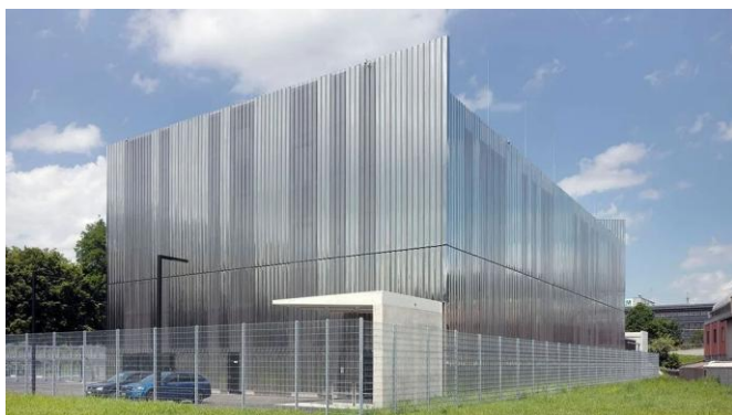
NorthC Datacenter in Biel
